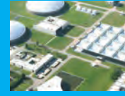
Drinking Water Treatment
