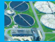
Urban Sewage Water
